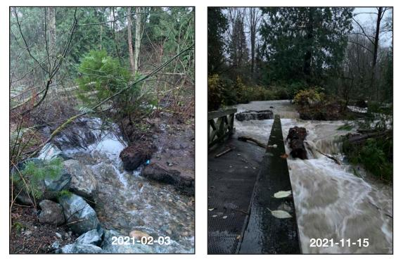
Subsequently, the City placed large boulders on one side of the new channel in an attempt to prevent erosion of the Trail and protect two large cedar trees standing near the bridge.
